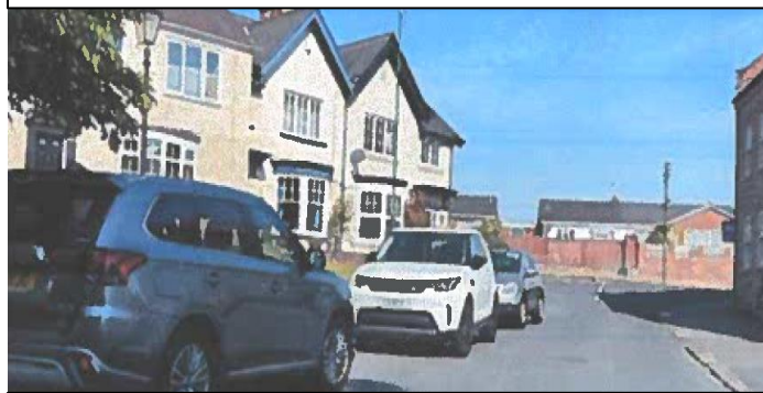
Carriageway can accommodate one-side of on-street parking only.
